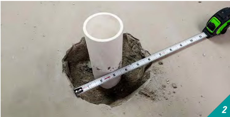
2 Begin breaking the concrete around the waste pipe to produce a hole that is roughly 5 ½" to 6 ½" in diameter, around waste pipe. The hole should be centered with the waste pipe. Use a tape measure to ensure the hole size is within the range, measuring in several locations.
