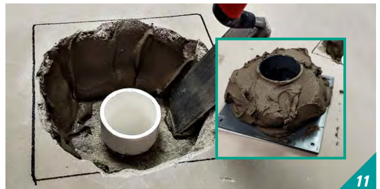
Using a margin trowel, apply modified thin set mortar around the outside perimeter of the hole leaving enough space for application of PVC cement (or ABS). Apply modified thin set mortar to the drain body such that the mortar approximates the volume of the hole around waste pipe. Use excess mortar so that it will squeeze out as the drain is installed. Modified thin set mortar with peanut butter consistency works best to prevent sag. Make sure waste pipe and drain body bonding surfaces are clean.
