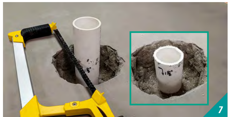
Using a hack saw or other means, cut the PVC waste pipe above the floor elevation mark. To prevent debris from entering the waste pipe, stuff a cloth inside the pipe below the cutting area. Once the cut is complete, vacuum debris and remove cloth.
