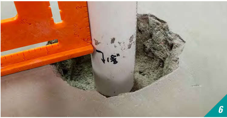
Using a speed square and permanent marker, mark the exact slab elevation on the pipe.
