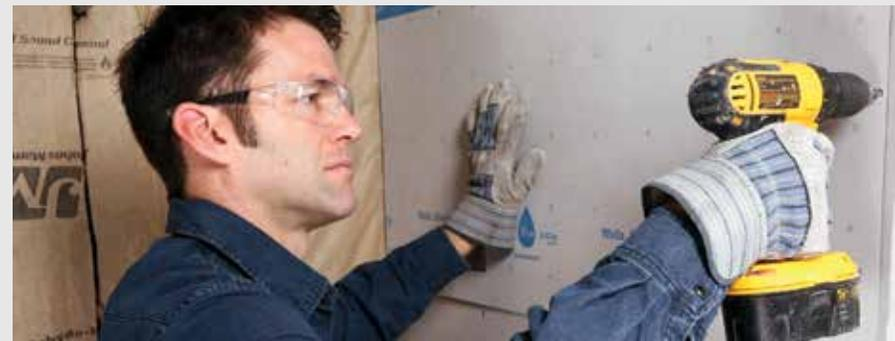
**NOTE:** Make sure your fasteners are flush with the surface of the GoBoard.
