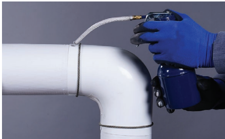
3. After the fitting cover has cured at least 10 minutes, run a bead of adhesive along its circumferential edge. Overlap the fitting cover (by approximately 1" [25 mm]) with a section of Zeston PVC jacketing and secure the circumferential joint with an elastic cord. The cord may be removed after approximately 10 minutes.
