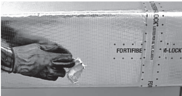
Damage to duct wall
