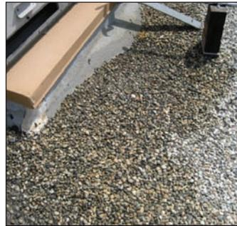
Some roofs have areas without positive drainage or slope, especially in older constructions. When installing a JM BUR roofing system with PermaMop asphalt, a ponding water rider will cover roofs with negligible slope [no less than 1/8" in 12" (10 mm/m) slope] and/or intermittent areas of ponding water. Johns Manville defines intermittent areas of
