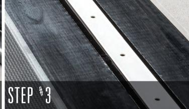
Set the batten strip on top of the exposed tape along the length of the seam.
