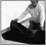
7. To install a parallel cap sheet, pick up a relaxed sheet and align it on the 8" (203 mm) selvage of the previously installed utility sheet.
