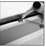
2. To use *JM*CleanBond Utility Sheet as a valley starter sheet, position the utility sheet so that it is centered down the middle of the drain, leaving the plastic release film adhered. Note: The base sheets should already be installed so the seam of the finished side lap is centered down the drain and will be centered under the utility sheet. The sides of the utility sheet should align with the perforation down the centers of the two base sheets.
