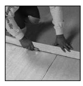
**10.** To install a cap sheet perpendicular to the utility sheet, pick up a relaxed sheet and position it so the end aligns with the 8" (203 mm) selvage of the installed utility sheet.
