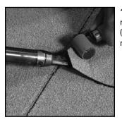
**18.** End laps must be rolled with a rounded edge roller and a ½" (3 mm) bleedout of SBS compound is required.
