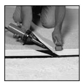
**16.** Once the cap sheet is installed, special care must be taken to heat sink the granules with a hot air gun for all end lap areas. Note: MBR® Flashing Cement or MBR® Utility Cement can be substituted for heat welding.
