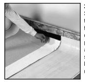
**3.** To use *JM*CleanBond Utility Sheet as a header sheet, begin at the lowest point on the roof. Lay in a full-width piece of the utility sheet over the already installed base ply, leaving the plastic release film adhered for both the base and utility sheets. Note: The base sheet side lap should be centered under the utility sheet.
