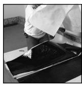
**4.** Fold the utility sheet in half along its length and strip off the leading half of its plastic film and the matching plastic film from the base sheet.
