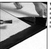
**17.** Prepare the end lap by removing all loose granules. With a hot air gun, apply heat to the 4" (102 mm) end lap area making sure both sheets have a good compound flow to adhere the two surfaces.
