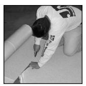
**1.** Cut *JM*CleanBond Utility Sheet and *JM*CleanBond<sup>®</sup> Cap Sheet to usable lengths and set aside, allowing them to relax. Make certain that the *JM*CleanBond<sup>®</sup> Base ply is clean and dry and that the ambient temperature is 45°F (7°C) or higher.
