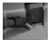
2. Where necessary, prepare surfaces using a grinder or other suitable means.
