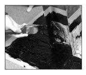
**9.** Apply a light coating of MBR Flashing Cement.
