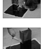
**12.** After drying, remove masking tape.
