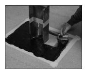
Coat the masked off area with a very thin coating [30 mil (0.76 mm)] of MBR Flashing Cement. A brush works best.
