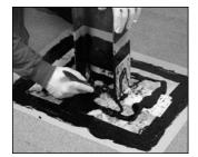
Re-coat the entire masked off area with a thicker [60 mil (1.52 mm)] coating of MBR Flashing Cement.
