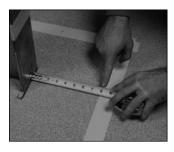
5. Precut the first piece of PermaFlash Scrim. Start 6" (152 mm) above the roof surface and extend fingers 6" (152 mm) onto the roof surface. PermaFlash Scrim is 12" (305 mm) wide for ease of application.
