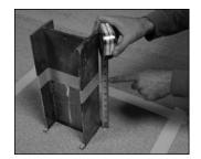
4. Use tape to mask off the top of the detail 8" (203 mm) above the roof and an 8" (203 mm) perimeter surrounding the detail.
