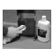
Prime the penetration with a light coating of PermaFlash Primer. A rag or spray bottle works best; a brush may apply too liberally.
