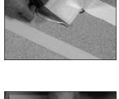
6. Precut the second piece of PermaFlash Scrim to serve as a target piece laying flat on the roof surrounding the penetration. Extend a minimum of 6" (152 mm) on the roof surface in all directions.
