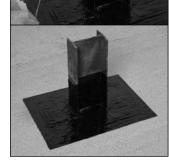
Completed Detail. 1/2 cartridge of MBR Flashing Cement used to complete detail.
