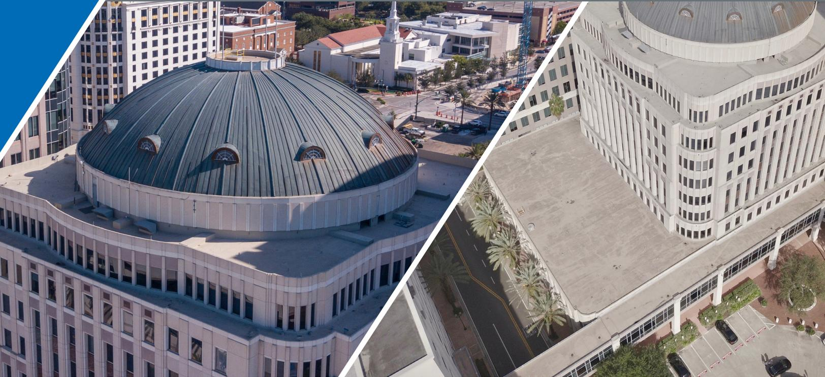
**Description:** 25 years after construction, Orlando's City Hall roof needed to be evaluated for replacement or restoration. Through extensive research, including moisture survey testing, it was determined that restoring the existing roof was the most efficient approach for this seven-level, nine-story downtown showcase.
