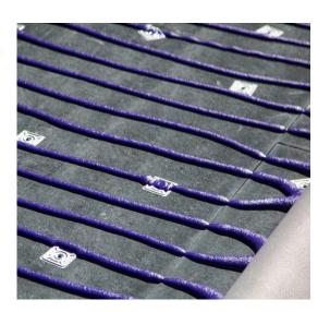
\*Green strength can be defined as the bond strength of an adhesive before it has fully cured and reached its final ultimate tensile strength. This strength is usually considerably lower than the final ultimate bond strength.
