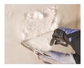
The PresSure Gauge is marked "2x4" on one side and "2x6" on the other. Use whichever marked side corresponds to the wall framing, pointing upward.
