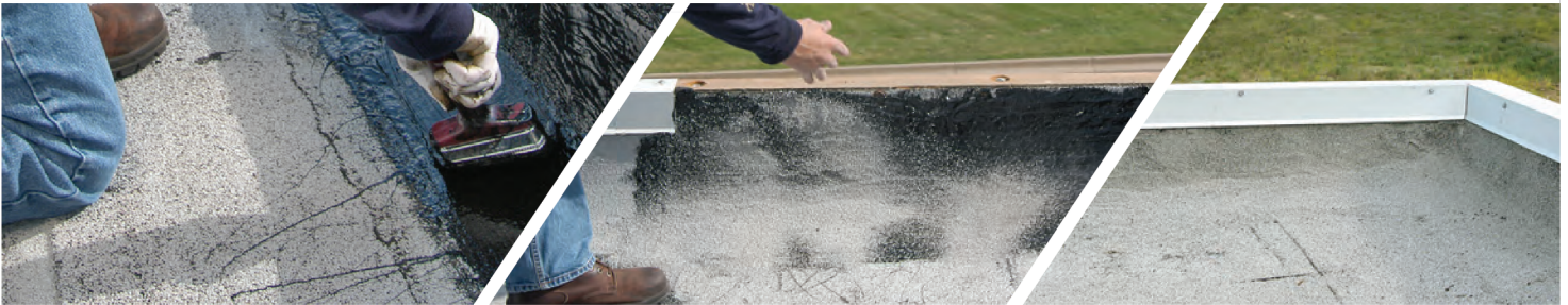
4. Coat entire scrim area
