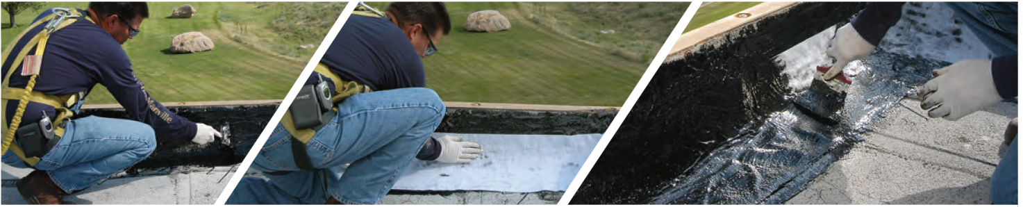
1. Apply base coat
