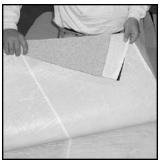
2. Begin at the lowest point on the roof and lay in a full-width sheet of JMCleanBond Cap over the JMCleanBond Base, leaving the plastic release film adhered for both the base and cap sheet. Note: The base sheet side lap should be centered under the cap sheet.
