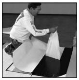
8. Fold the cap sheet in half along its length. Remove the plastic film from the leading half of the bottom of the new cap sheet, the top of the installed base sheet, and the selvage of the already installed cap sheet. Slowly lower the cap sheet into place taking care to keep it aligned and free from wrinkling.
