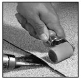
13. End laps must be rolled with a rounded edge roller and a  $\frac{1}{8}$ " (3 mm) bleed-out of SBS compound is required.
