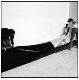
3. Fold the cap sheet in half along its length and strip off the leading half of its plastic film. Next, strip off the matching plastic film from the base sheet.
