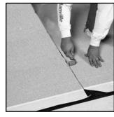
**12b.** Set the lap in place, and roll with a hand roller.
