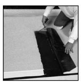
3. T-laps can also be seated with a smooth coating of MBR Utility Cement in the triangle of the lap Note: Backwater Laps
