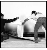
**5.** Fold back the other half of the cap sheet and repeat the steps used for installing the first half of the sheet.
