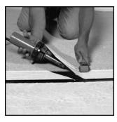
11. Once the cap sheet is installed, special care must be taken to heat sink the granules with a hot air gun for all end lap areas. Note: MBR® Flashing Cement or MBR® Utility Cement can be substituted for heat welding, if required.
