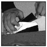
10. Note: Where two sheets come together at the end laps, score and leave a 4" (102 mm) piece of release film on the bottom of the overlapping sheet's end lap area. This will reduce the chance of the sheet adhering to the granules of the lower sheet.
