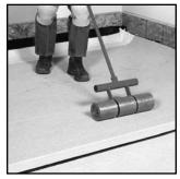
**14.** After all cap sheets are installed, roll across the width of the sheet first, then across its length with a 75 lb to 100 lb (34 kg to 45 kg) split-wheel, weighted roller to set the cap sheets, paying special attention to the selvage seams.
