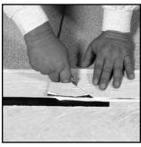
7. Where a "T" joint exists, cut off the corner of the selvage at a 45° angle where the end overlaps the side lap of the previously installed cap sheet. This will reduce membrane thickness when the next sheet is applied.
