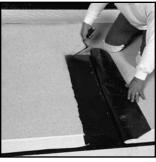
**12a**. Alternatively, apply a thin coat of MBR Utility Cement to the end lap area with a trowel.
