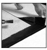
12. Prepare the end lap by removing all loose granules. With a hot air gun, apply heat to the 4" (102 mm) end lap area making sure both sheets have a good compound flow to adhere the two surfaces.
