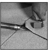
Use a hot air gun to weld the top lap to the bottom lap. Make sure both sheets have good compound flow.
