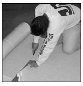
1. Cut to usable lengths and set aside, allowing them to relax. Make certain that the *JM*CleanBond® Base ply is clean and dry and that the ambient temperature is 45°F (7°C) or higher.
