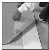
**6.** To install another cap sheet, pick up a relaxed sheet and align it on the 4" (102 mm) selvage of the piece already installed.
