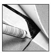
Apply a thin bead of cement along the diagonal side of the T-lap.
