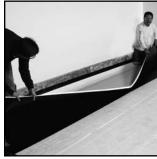
**4.** Lower the cap sheet slowly onto the base sheet, from the center out.
