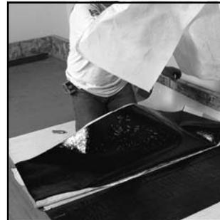
4. Fold the utility sheet in half along its length and strip off the leading half of its plastic film and the matching plastic film from the base sheet.
