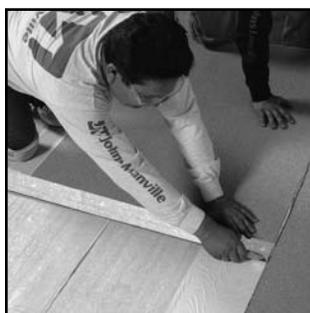
**11.** Holding the cap sheet in position and using its sides as a guide, score the plastic release film at the end of the base sheets below, so that you will be able to remove only those portions of release film that are directly under the cap sheet. You will also need to score the sides of the release film on the selvage of the utility sheet where the cap sheet overlaps it.
