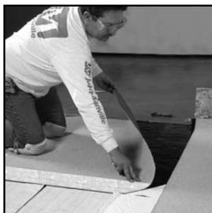
**13.** Fold the cap sheet in half along its length. Remove the plastic film from the leading half of the cap sheet, the top of the installed base sheet, and that portion of the utility sheet selvage that is directly under the cap sheet. Slowly lower the cap sheet into place taking care to keep it aligned and free from wrinkling.
