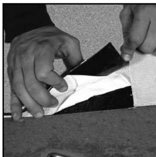
**15.** Note: Where two sheets will come together at the end laps, score and leave a 4" (102 mm) piece of release film on the bottom of the overlapping sheet's end lap area. This will reduce the chance of the sheet adhering to the granules of the lower sheet.
