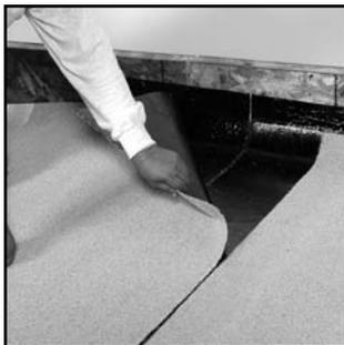
**8.** To install a cap sheet parallel to the utility sheet, fold the cap sheet in half along its length. Remove the plastic film from the leading half of the cap sheet, the top of the installed base sheet, and the selvage of the installed utility sheet. Slowly lower the cap sheet into place taking care to keep it aligned and free from wrinkling.
