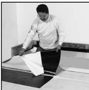
**14.** Fold back the second half of the cap sheet, remove its plastic film and the matching film portion from the base sheet and utility sheet selvage. Slowly lower it into place from the center out.
