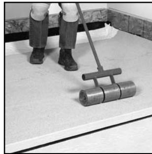
**19.** After all cap and utility sheets are installed, roll across the width of the sheet first, then across its length with a 75 lb to 100 lb (34 kg to 45 kg) split-wheel, weighted roller to set the cap sheets, paying special attention to the selvage seams.
