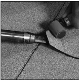
**18.** End laps must be rolled with a rounded edge roller and a 1/8" (3 mm) bleedout of SBS compound is required.
