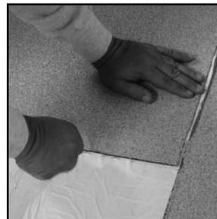
7. To install a parallel cap sheet, pick up a relaxed sheet and align it on the 8" (203 mm) selvage of the previously installed utility sheet.
