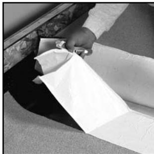
**9.** Fold back the second half of the cap sheet, remove the plastic film and the matching film portion from the base sheet. Slowly lower it into place from the center out.
