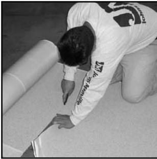
1. Cut JM CleanBond Utility Sheet and JM CleanBond® Cap Sheet to usable lengths and set aside, allowing them to relax. Make certain that the JM CleanBond® Base ply is clean and dry and that the ambient temperature is 45°F (7°C) or higher.
