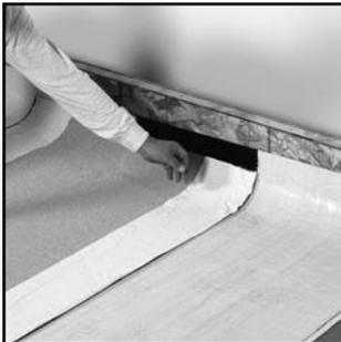
3. To use JM CleanBond Utility Sheet as a header sheet, begin at the lowest point on the roof. Lay in a full-width piece of the utility sheet over the already installed base ply, leaving the plastic release film adhered for both the base and utility sheets. Note: The base sheet side lap should be centered under the utility sheet.
