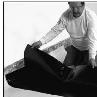
6. Fold back the other half of the utility sheet and repeat the steps used for installing the first half of the sheet.
