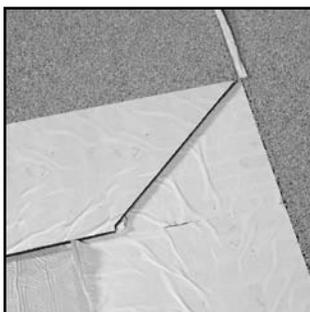
**12.** To execute a proper "T"-joint, cut off the corner of the cap sheet selvage where the end overlaps the selvage of the utility sheet. This will reduce membrane thickness when the next sheet is applied.
