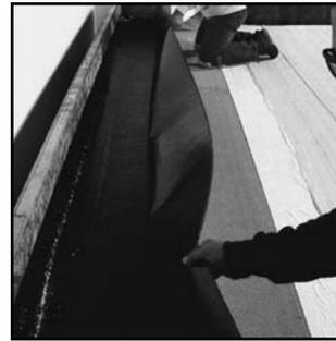
2. To use JM CleanBond Utility Sheet as a valley starter sheet, position the utility sheet so that it is centered down the middle of the drain, leaving the plastic release film adhered. Note: The base sheets should already be installed so the seam of the finished side lap is centered down the drain and will be centered under the utility sheet. The sides of the utility sheet should align with the perforation down the centers of the two base sheets.
