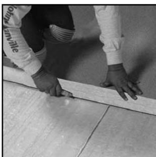
**10.** To install a cap sheet perpendicular to the utility sheet, pick up a relaxed sheet and position it so the end aligns with the 8" (203 mm) selvage of the installed utility sheet.
