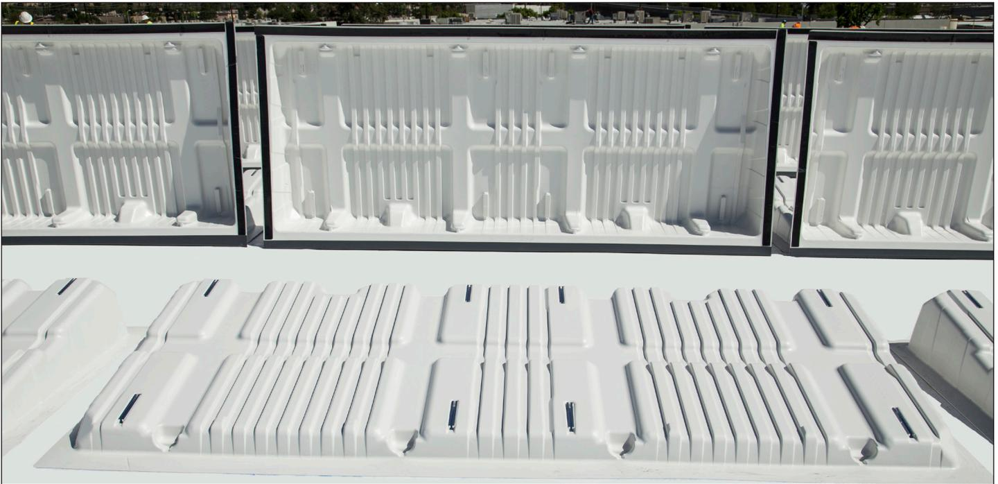
Carefully lower the ENERGY Curb unit back into position on the roofing surface and use a 10 lb (4.54 kg) weighted roller to apply pressure to the topside of the flanges.
