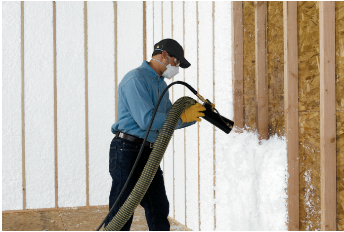
JM Spider® spray-in fiber glass insulation provides superior energy efficiency and noise control.
