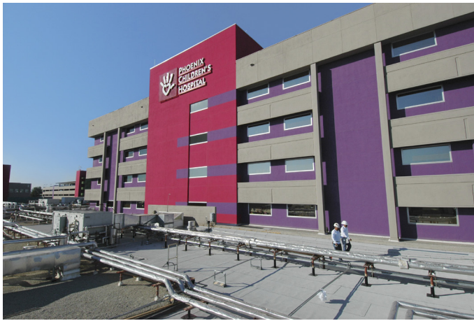
JM's roofing system protects the post-operative care unit of this Children's Hospital in Phoenix.
