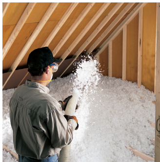
Blow-in Formaldehyde-free™ fiber glass insulation is ideal for maintaining thermal performance for the life of the home.
