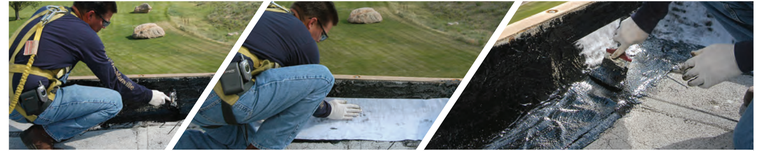
1. Apply base coat
