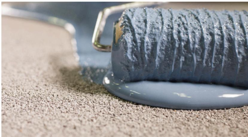
JM Coating Universal Base should be applied in the morning hours to allow maximum cure time. Temperatures shall be above 55°F (12°C) and rising, but not above 110°F (43°C) ambient. Do not apply if rain or freezing temperatures are predicted within 24 hours. Excessive heat can cause flash drying, thus it is not recommended for application to surfaces 140°F (60°C) or greater.
