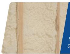
Lower-density, nonstructural, opencell SPF delivers the highest yield of any JM Corbond open-cell product.
